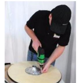
Fasten the coupler to the table top with the 6 screws.
